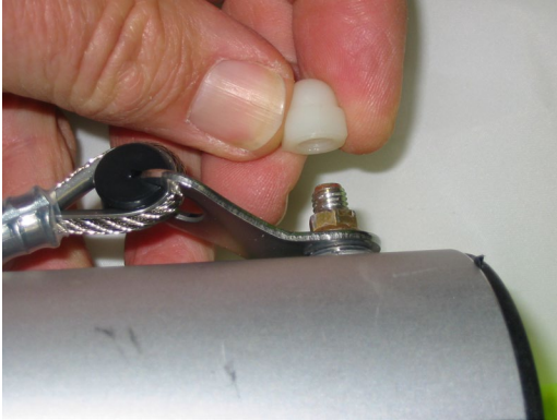
Installation of clinch nut
